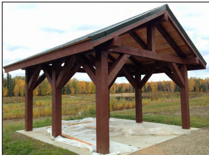
Canon Cogan partnered with Alaska State Parks to complete his Eagle Scout community service project. Canon and Troop 1001 logged over 600 hours of volunteer service constructing a picnic shelter at Olnes Pond in Lower Chatanika River State Recreation Area.
