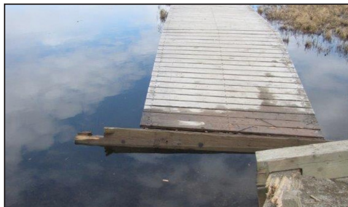
Winter takes its toll on parks in the Northern Area. This past winter, ice took out the dock at Lost Lake Campground in Quartz Lake State Recreation Area. Northern area maintenance staff will have the dock repaired within the month.
