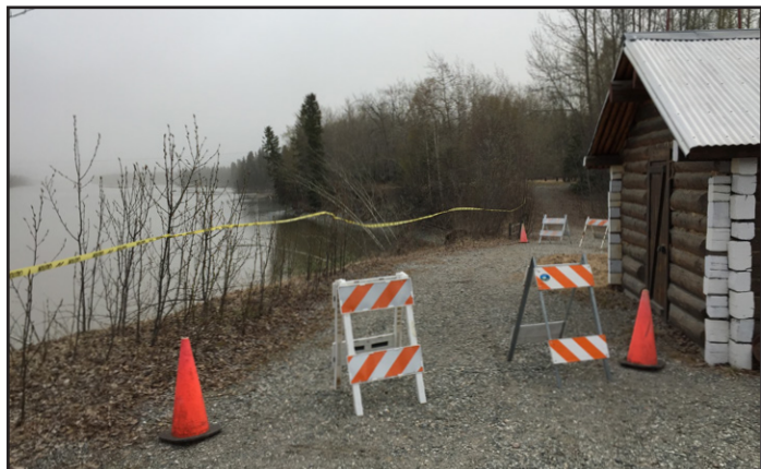
The mighty Tanana River is threatening historic structures at Big Delta State Historical Park. Extreme erosion, due to the sudden release of an ice jam this spring, encroached within 23 feet of the Billy Mitchell Cabin, also known as the Military Residence. Chief of Design and Construction Rys Miranda and Engineering Manager Luke Randall visited the site in mid-May to assess the situation and develop a plan of action to stabilize the river bank and protect the historic structures near the river.
