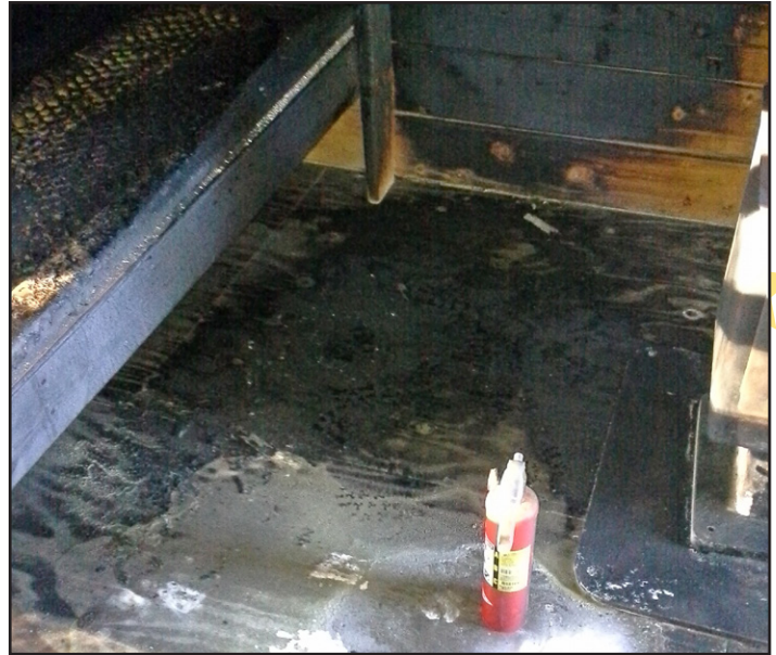
Damage to the cabin was extensive, even with the use of a fire extinguisher.
