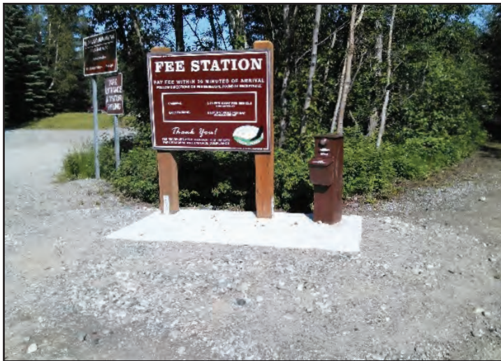
As part of Alaska State Parks commitment to becoming more self-sufficient, day-use parking fees are now being charged at Big Delta State Historical Park and Lower Chatanika State Recreation Area. Northern Area maintenance staff installed this fee station sign at Big Delta State Historical Park this spring.
