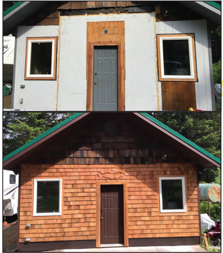
The Lowell Point SRS bunkhouse exterior before and after renovation
