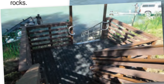
Lower level deck of newly installed river access stairs
