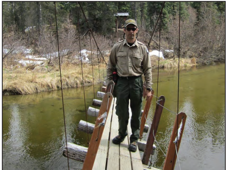
Specialist Chris Love (now ranger) on Byers Creek Bridge in 2013, before re-tensioning the cables.
