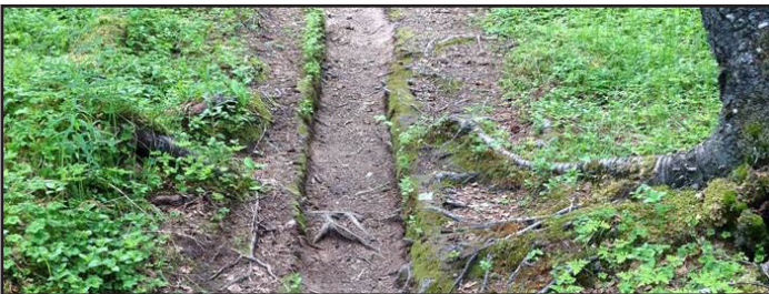
Little Coal Creek Trail's well-worn, rutted tread before work
