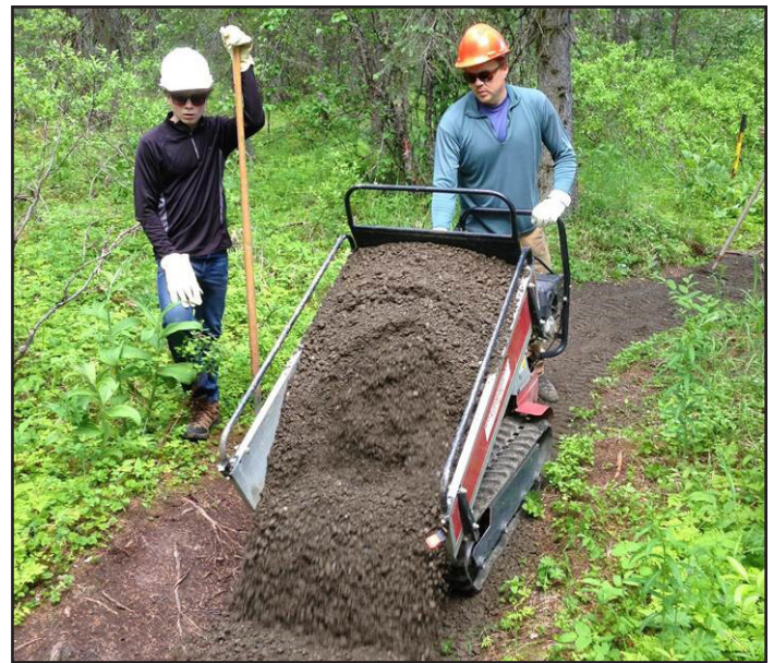
YCC crew leader Rob Shelby and worker John Hicks move and spread gravel with a powered wheelbarrow.
