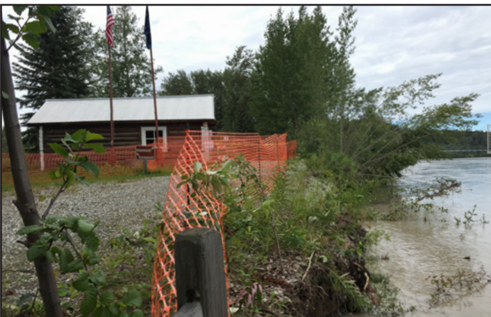
The closest building to the river, which was 14 feet from the bank, was moved to protect the structure. This move also provided room for a crew from the Office of History and Archaeology to work on the riverbank, recovering artifacts before they are lost to riverbank erosion.
