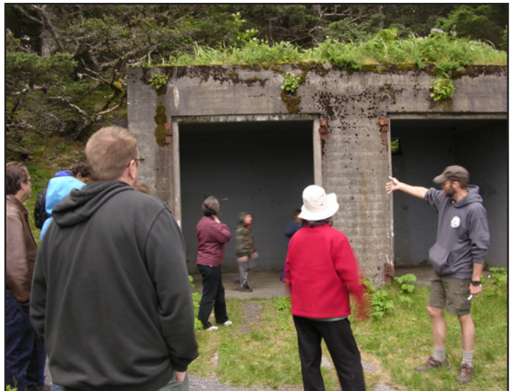
This searchlight bunker, when restored, is the planned home for the new searchlight.
