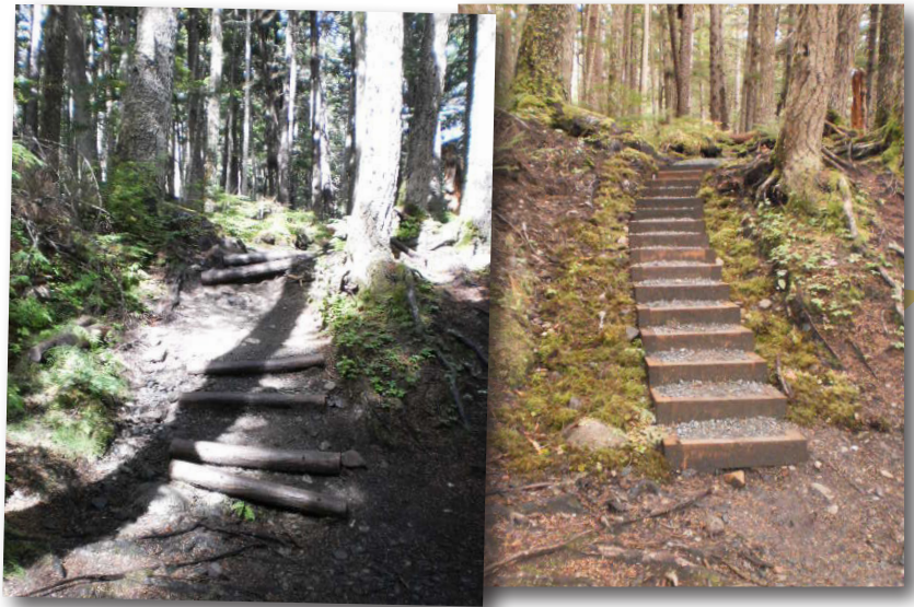
These before and after photos show dilapidated log steps and newly constructed pressure-treated crib steps.
