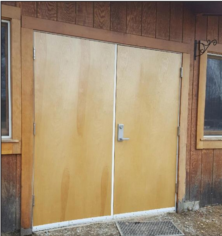
New doors installed at Rika's Café and Gift Shop
