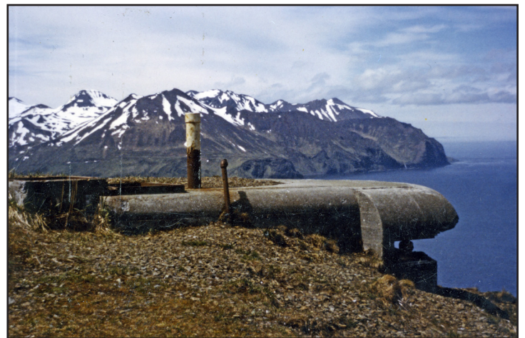
Photo taken by Paul Chattey. It is entirely within the range of possibility and coincidence that Tim Smith is the person looking out of the observation slit. Location was Ulatka Head on Mount Ballyhoo above Dutch Harbor, this was one of the battery command observation posts in the harbor defenses.
