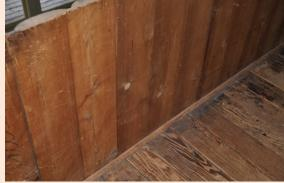
at the floor boards. Each piece of siding is attached by four nails. Quarter round finishes the wall on the loft side. Evidence that the pony wall is pulling away from its vertical orientation is seen near each wall. This attachment method creates an unstable wall and a safety concern.
